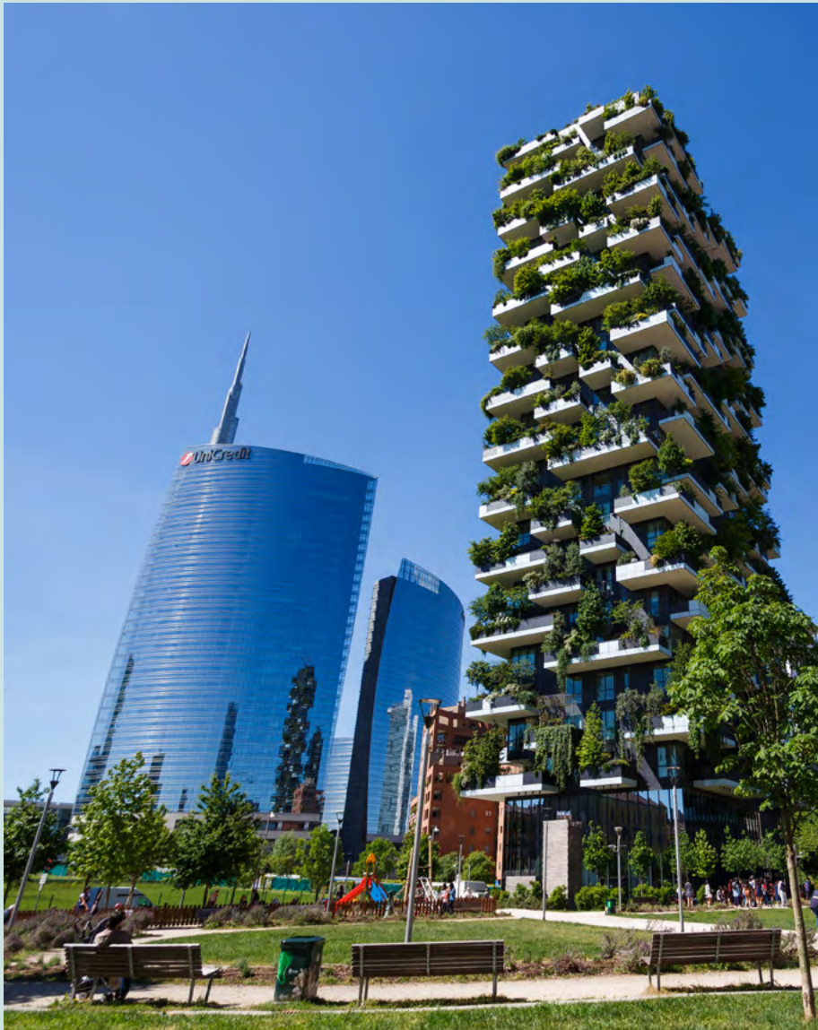
Italy: Bosco Verticale (Vertical Forest) sustainable architecture in Porta Nuova district, in Milan.
